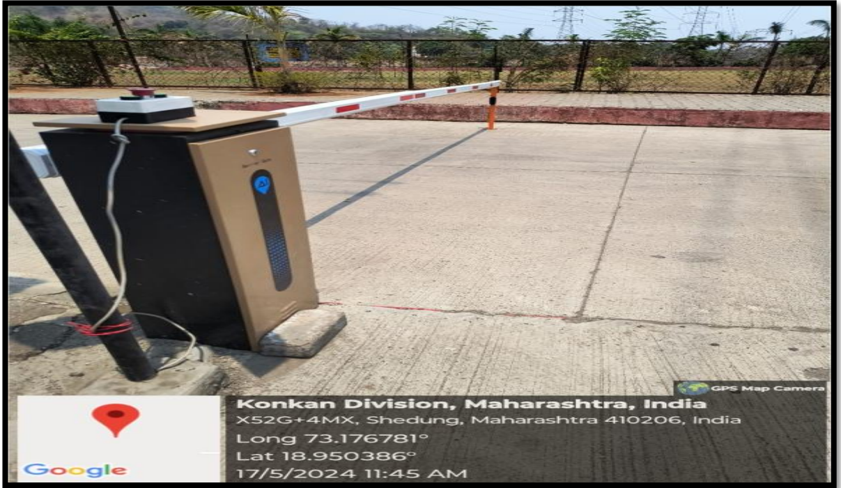
Road Safety Barrier
